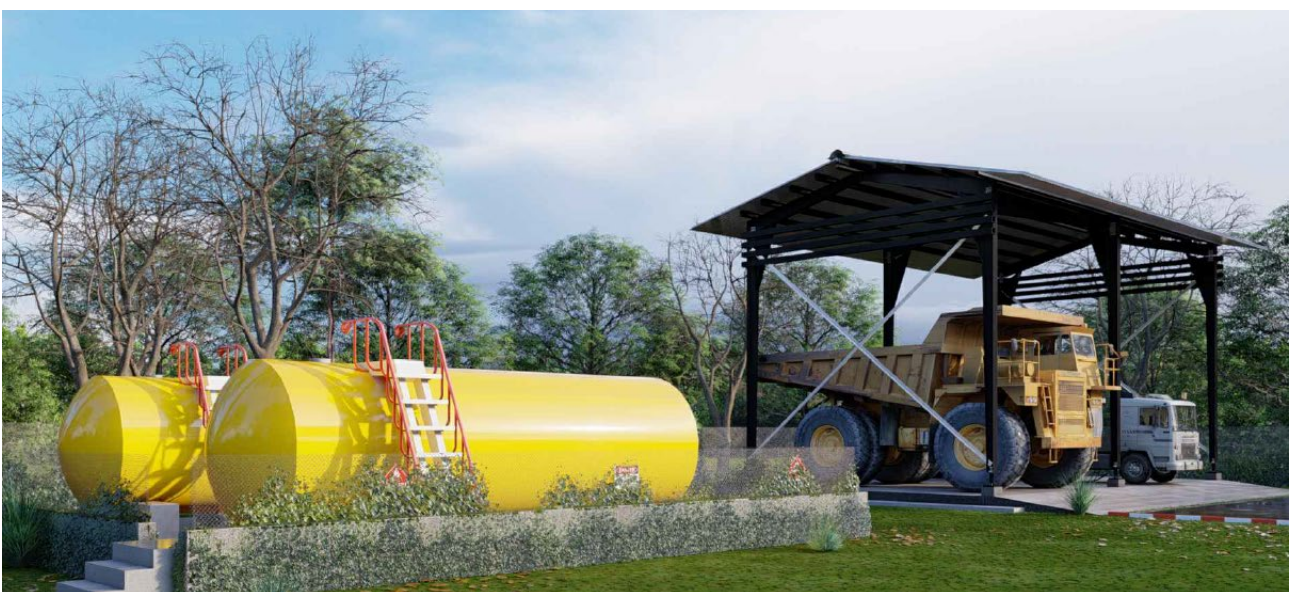
Figure 10. 3D rendered image of the fuel farm which includes two 40,000-litre bulk fuel storage tanks
