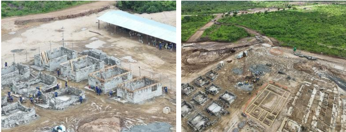
Figures 11 & 12. Progress at the site camp facilities, showing completed foundation excavations, construction of VIP accommodation units, and advancement of Mess Hall, BQ accommodation and entrance earthworks supporting upcoming project mobilisation
