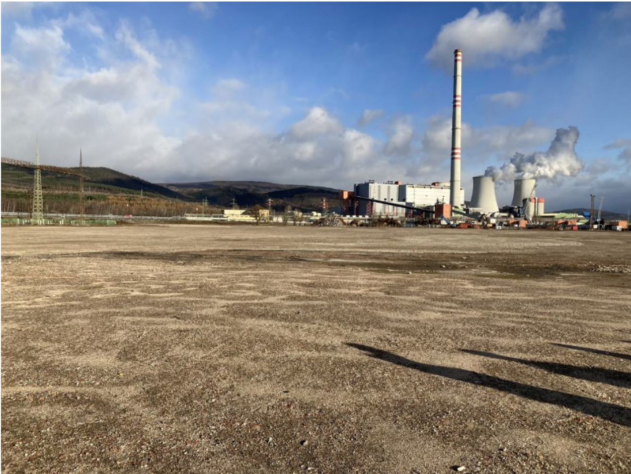
Figure 11-2: Pruněřov Site following Demolition of EPR 1
