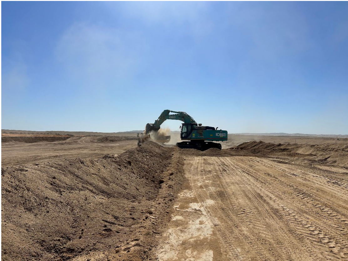
Figure 4: Excavation of Counter Current Decantation (CCD) area foundations.
