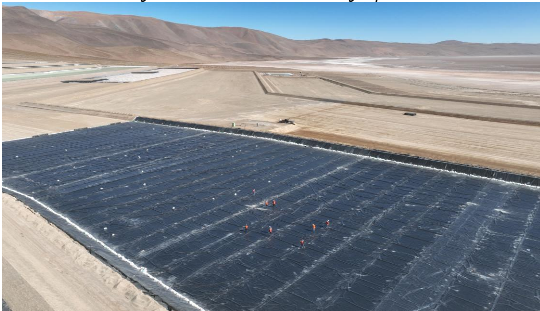
Figure 3. Liner installation team working on pond 4
