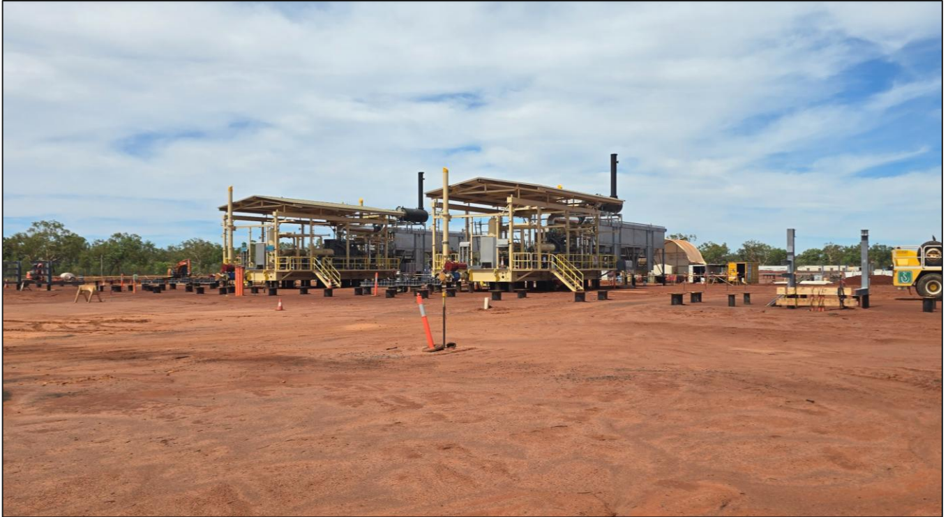
Figure 2 – Compressor units installed on SS2 pad
