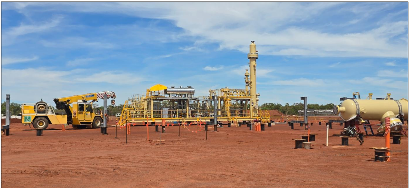
Figure 3 – TEG package installed on SS2 pad
