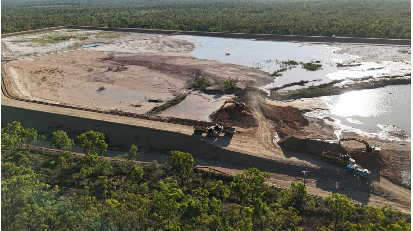
Figure 3: 10 th Layer (Final) In progress with downstream lift and final upstream lift for Lot 1 and Lot 6
