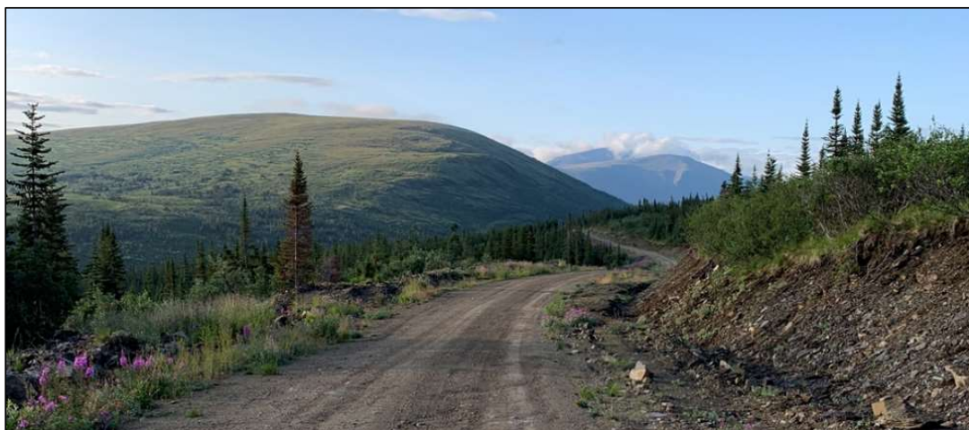
Figure 2-3: View of the Tote Road (looking south towards the Process Plant and Mining Area) Source: BMC
