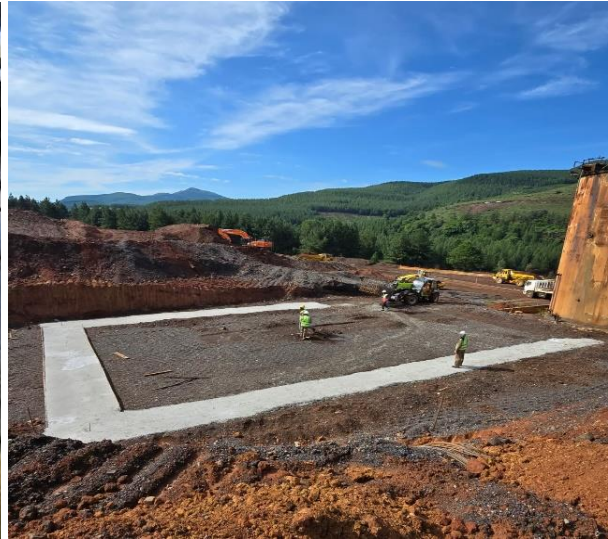
Figure 2: Blinding of the Gold Room's Foundations
