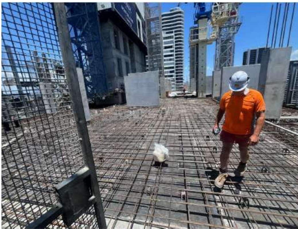
Level 16 eastern end with steel fixed. Western end is formed. Precast installed.
