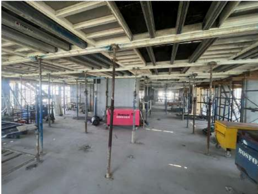
Level 15 - formwork to be stripped.
