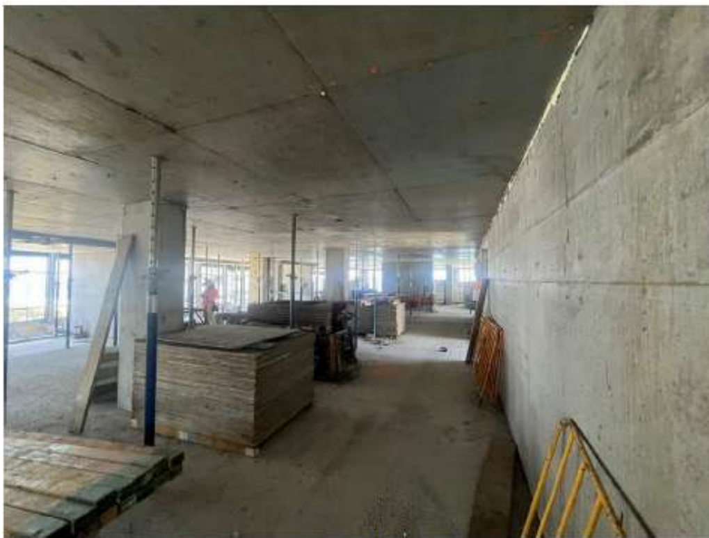
Level 14 – formwork stripped, ready for glazing.
