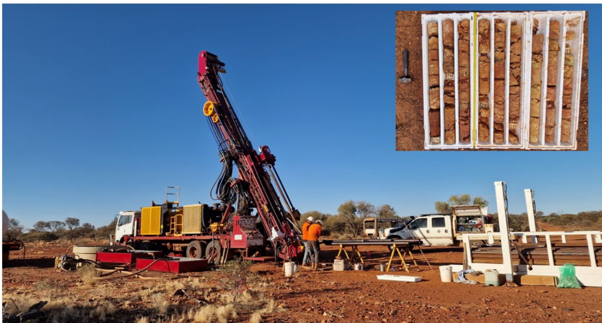
Figure 3 – Diamond rig drilling the wide diameter PQ core through near surface oxide and transition material. Inset picture shows examples of the PQ oxide core.
