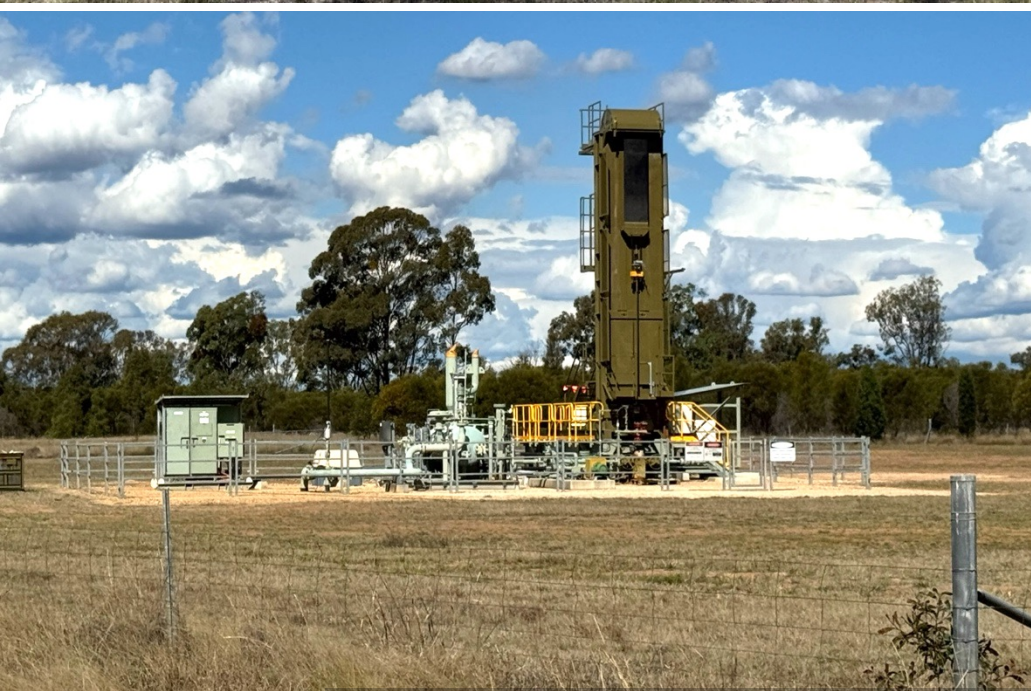
CSG Well – Origin Energy Well to South East of QBMC Project
