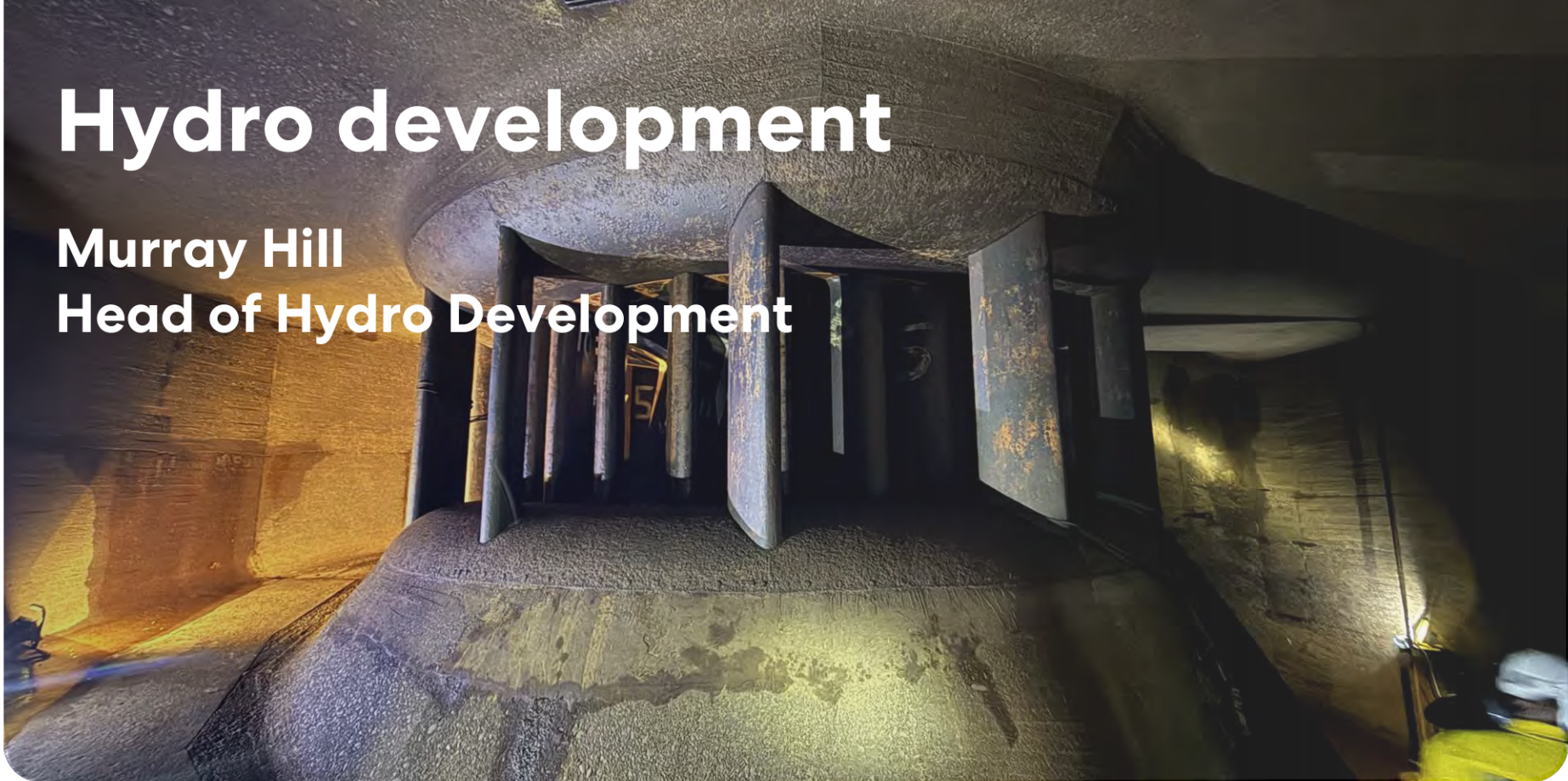
Waitaki Power Station – turbine inlet Unit 6.
