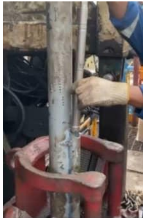
Completion Activity TE B01-003 installing PCP pump
