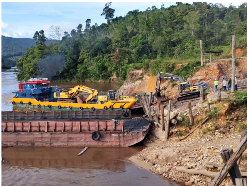
HML Fleet Unloading at Krajan Jetty
