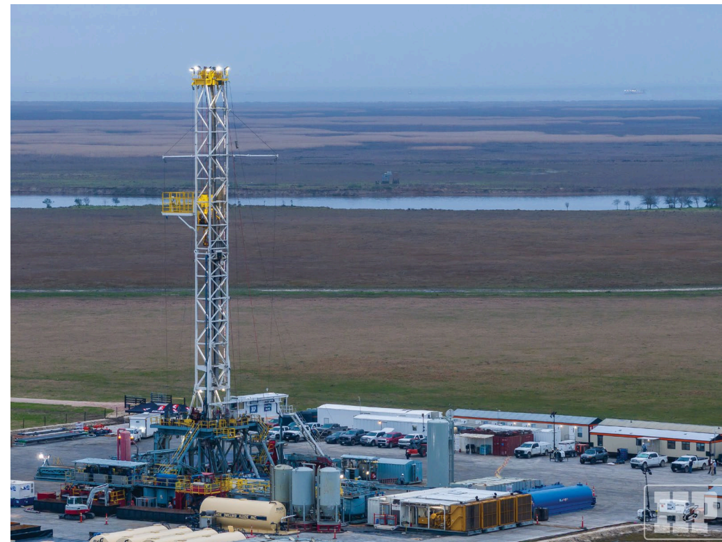
Representative drilling rig with similar specifications to the H&P 648 (FlexRigs®) planned for use in Omega's upcoming appraisal program. Vehicles located at the edge of the pad provide operation scale
