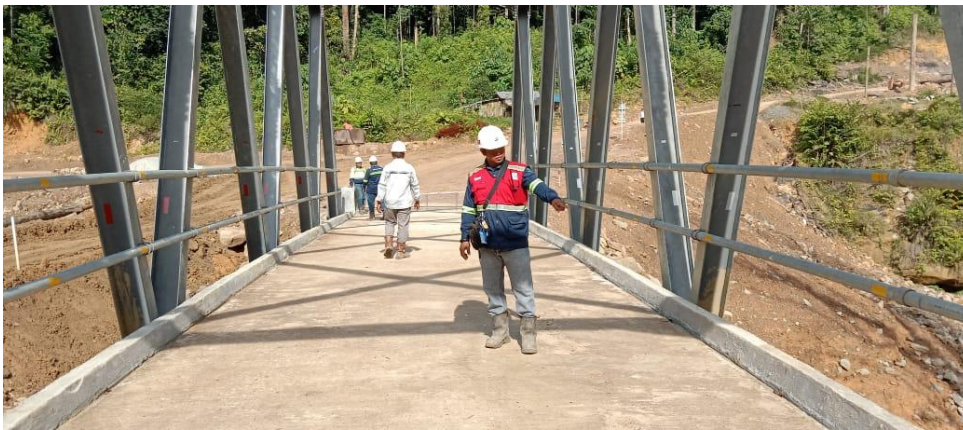
Mohing Steel Bridge Inspection
