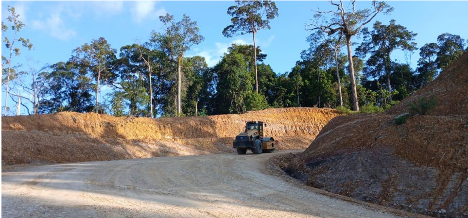
Haul Road Upgrade
