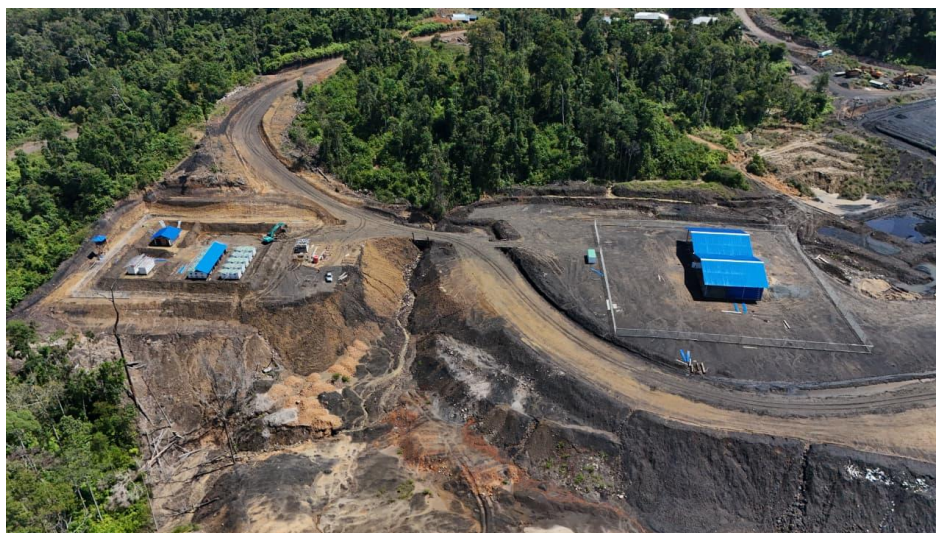
Drill and Blast Facilities
