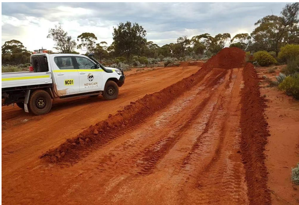
Figure 6: Drill pad clearing and earthwork in progress at Gimlet
