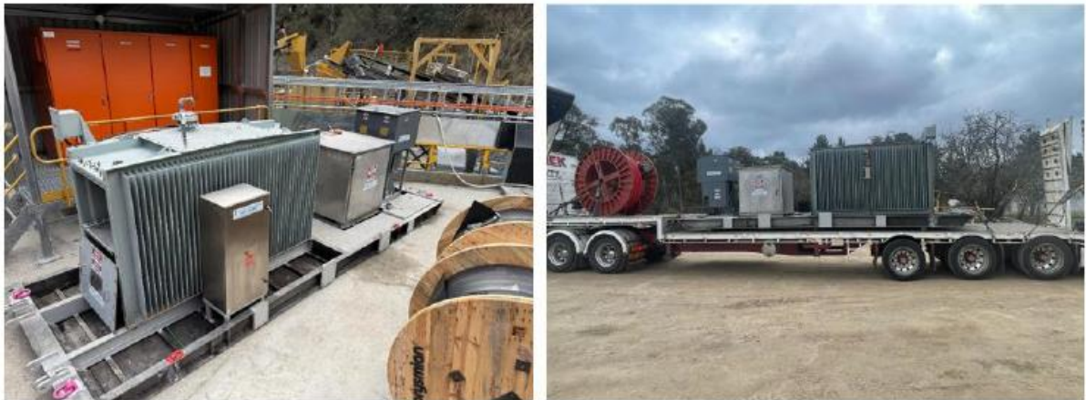
Image 2: High voltage (11 kV) transformer installed next to power station at the Reward Gold plant
