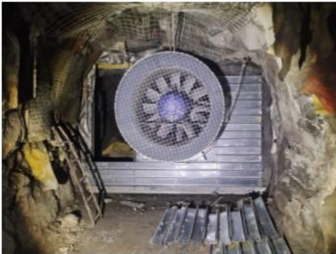
Image 8: Installation of 110kW ventilation fan
