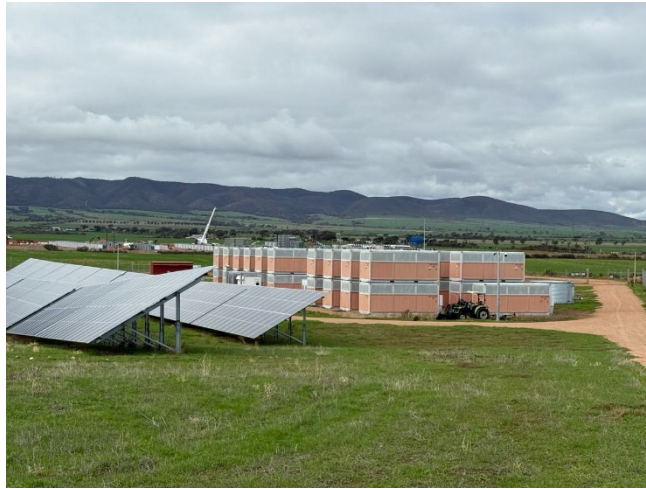
Yadlamalka solar and Invinty vanadium flow battery site (2MW/ 8MWhr)
