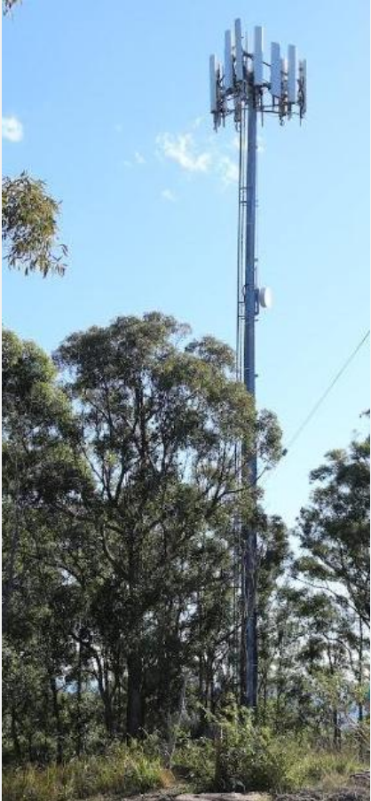
Securing mobile tower access
