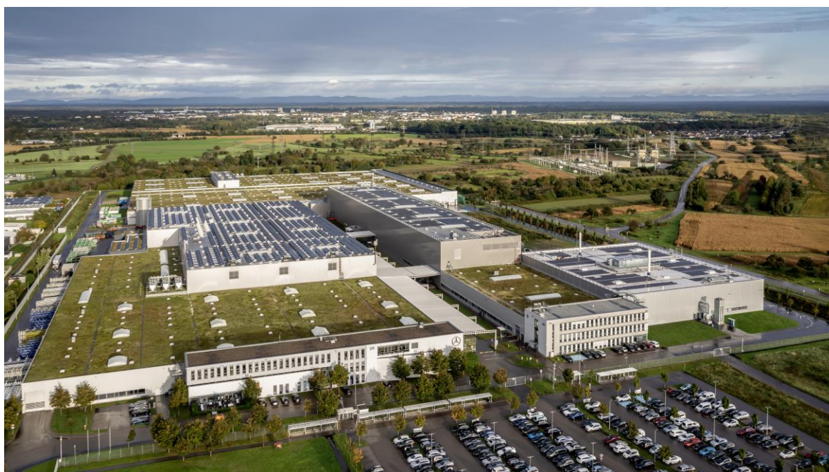
Figure 4 – Recycling Plant Building (far right) at Mercedes-Benz, Kuppenheim
