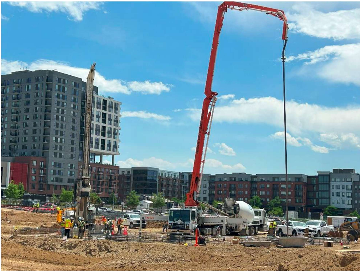
Figure 3. Pouring concrete for caissons
