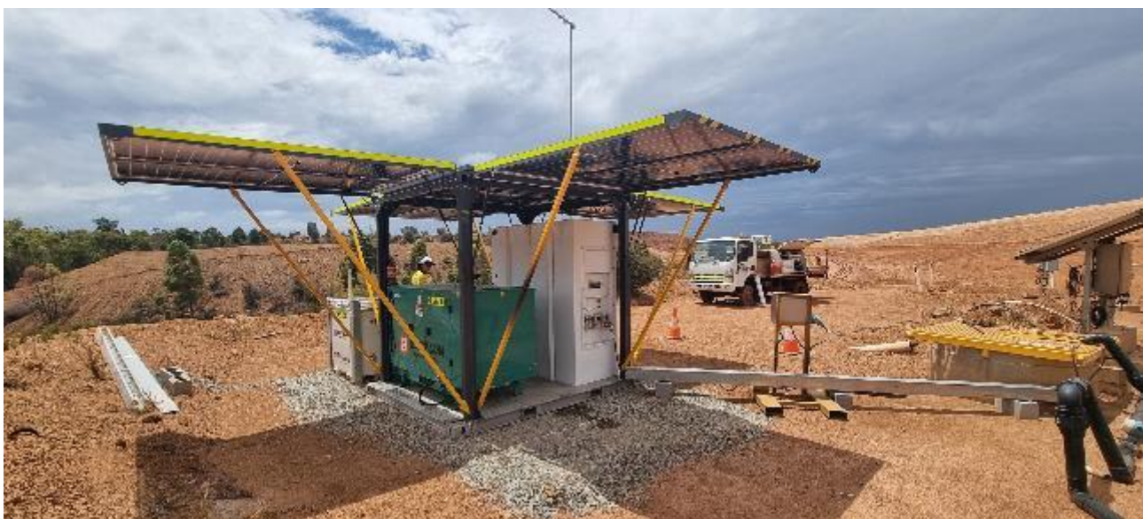
Installation and commissioning of a hybrid power unit
