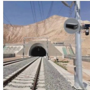
Installed over train tracks
